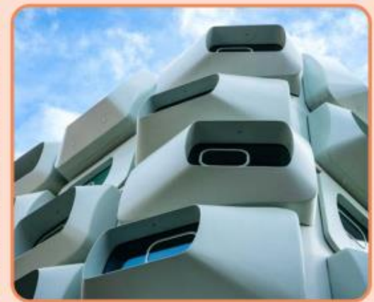
'Argos' building, Austria:
